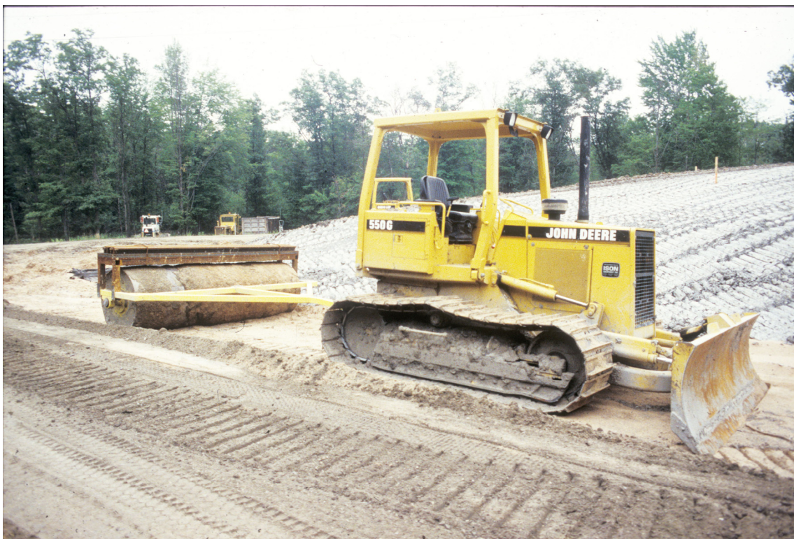
Figure 4.1 Residuals Placement with Low Track Pressure Dozer and Smooth Roller
