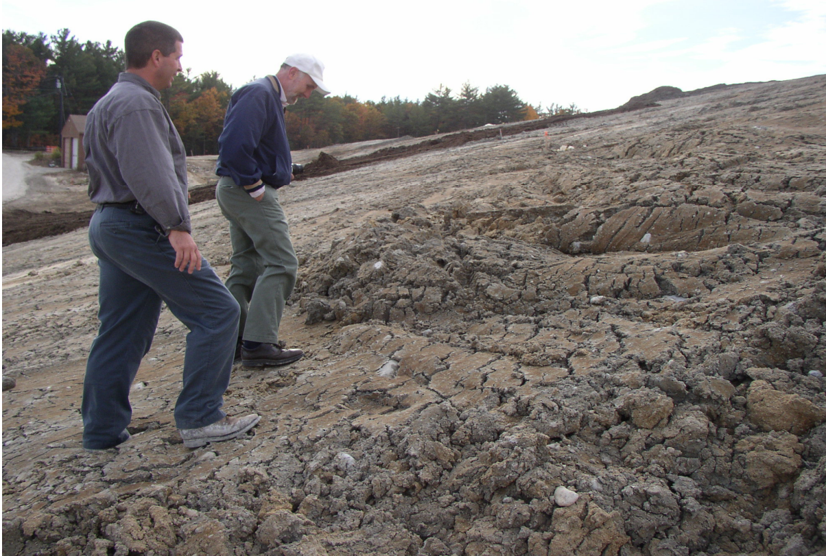
Figure 3.7 Slumped Area Due to High Moisture Content
