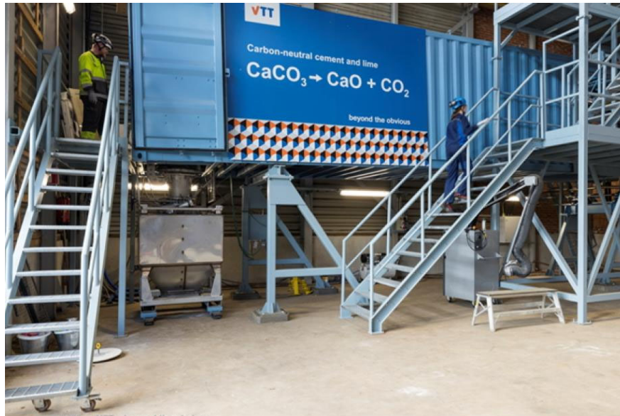
Figure 53. VTT's Electric Rotary Lime Kiln
