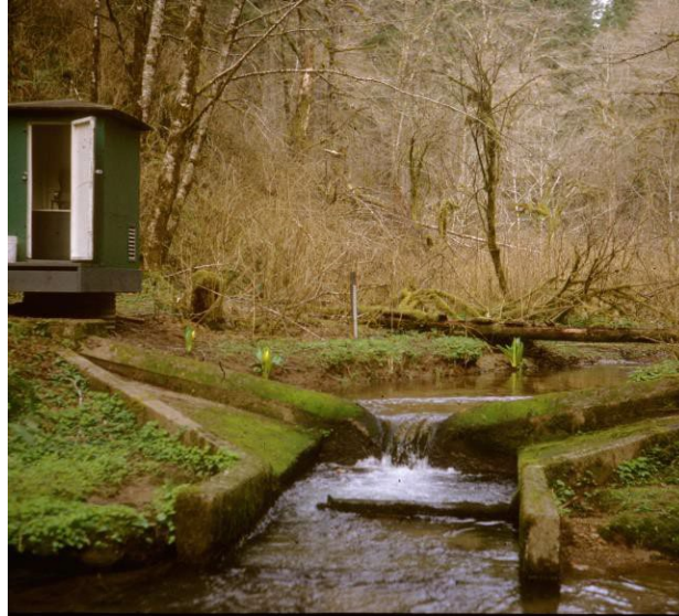
Figure B1. Broad-Crested Compound Weir at Flynn Creek and Outside Staff Gauge in Pool on River Right
