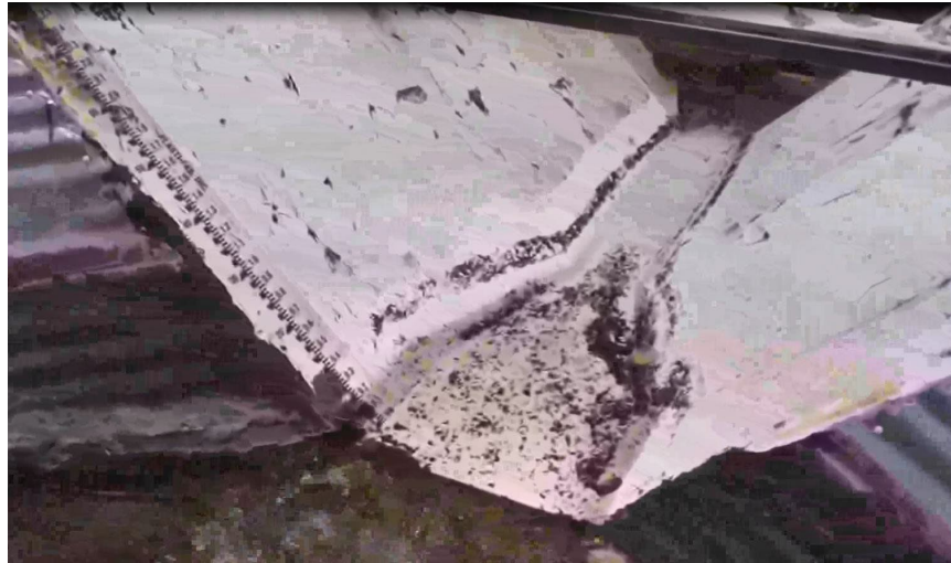
Figure B3. Trapezoidal Flume at NBU Gauging Station
